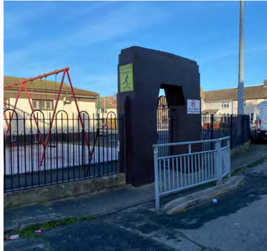
Entrance near Killane road with later additional safety barriers
